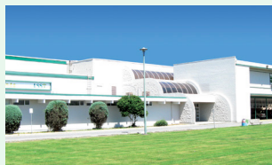
Langley Secondary (LSS)
